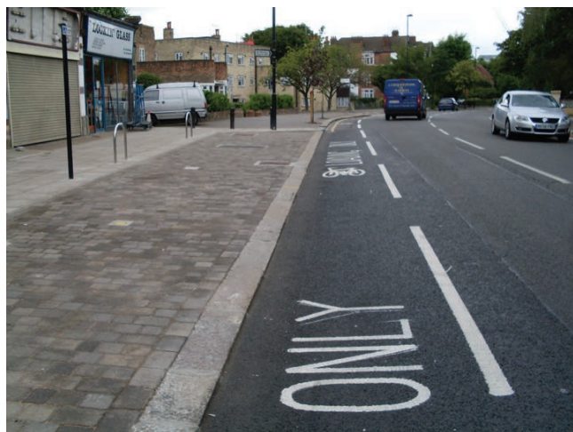
Figure 8. Inset parking bays. This photo shows a loading bay relocated to a wide footway in order to continue a cycle lane and reduce nearside conflict for passing cyclists. Repositioning parking bays may not be the most obvious cycling infrastructure asset but small measures like these can help improve comfort and safety for cyclists as they keep the road space and cycle infrastructure clear of blockages. This is referenced in the 2014 LCDS (TfL, 2014a) as nearside conflict. This scheme scores 49 on the cycling level of service assessment, which means it offers a good level of service. This route has no critical issues and helps resolve the issues associated with kerbside activity past loading bays
