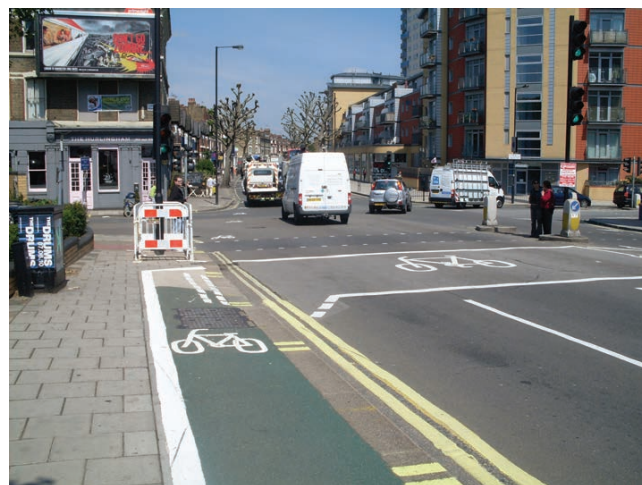
Figure 5. Cycle lane marked on the edge of the footway with transition back onto carriageway at 90° to traffic flow in an uncontrolled manner at a signalised junction. This photo shows that cyclists are asked to use the footway despite three general traffic lanes being present. This highlights the two approaches to designing for cyclists that engineers commonly use. Cyclists can be allowed onto pedestrian areas and advised to cross with pedestrians as a means of shielding them from conflict with motor vehicles (with larger mass and higher speeds) or cyclists can be recommended to take their place on the carriageway and behave as a vehicle mixed in with other vehicles. Transitions from one approach to another characterise delivery on LCN+, as evidenced by this photo. This inconsistency of approach is referenced as a major deterrent to cycling in the Mayor's vision for cycling (TfL, 2013). The cycling level of service assessment score is 29 out of 100, which means it offers a basic level of service. It has two critical issues – heavy streams of left-turning traffic cutting across the unprotected nearside cyclists and secondary position promoted where there is no space provided within the lane
