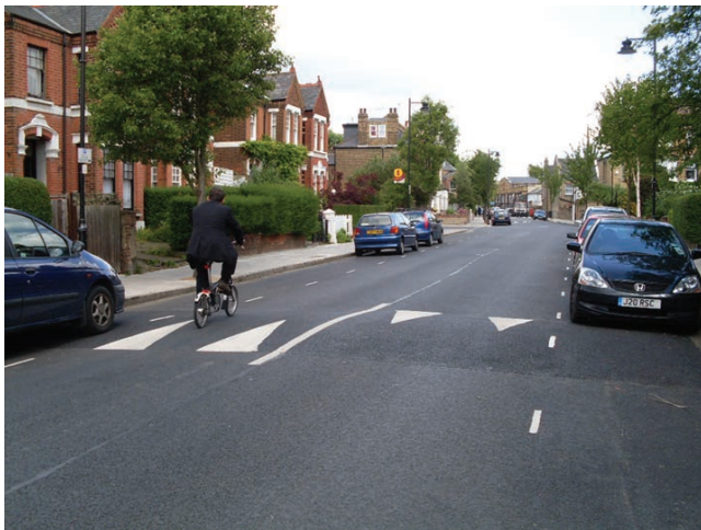
Figure 6. A speed hump with a sinusoidal gradual slope rather than a round-top hump presents a much smoother riding experience for cyclists without the impact of hitting the more vertical round-top profile. This was a key innovation brought in as part of the LCN+ project. The cycling level of service score is 72 out of 100, with the scheme scoring well in the ‘feeling of safety’ factors as it is a quiet back street route with traffic calming. This route offers the highest level of service despite the fact that no obvious cycling provision is in place
