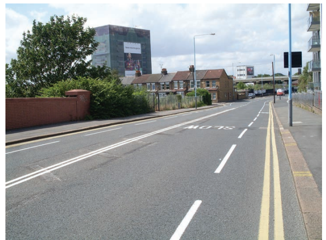
Figure 3. Cycle lane with associated parking restrictions, meaning it will be clear of traffic and so ensure a more consistent level of service to cyclists. When assessed using the cycling level of service, the scheme scores 40 out of 100, meaning it provides a good level of service. The main concern would be the feeling of safety as motor vehicle speeds are not calmed and the carriageway is wide and straight. This led to a critical issue as 85 percentile speeds exceed 30 mph (48 km/h). As a critical issue has been raised, the overall score is not relevant as the issue should be resolved in the design, either through traffic calming or a greater degree of segregation. The parking restrictions do mean that conflict with kerbside activity is minimised and this is a critical factor
