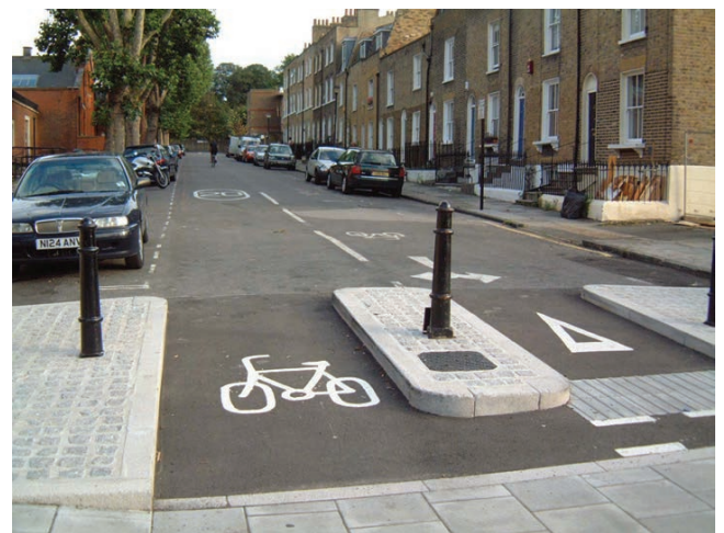
Figure 7. Point closure: road closed to general traffic but cyclists are allowed to move through. This effectively removes motorised through traffic, creating a pleasant, quiet and almost traffic-free situation (residents are still permitted to drive and park outside their properties). This scheme scores 76 out of 100 on the cycling level of service assessment, offering the highest level of service. It scores particularly well in terms of directness and feeling of safety
